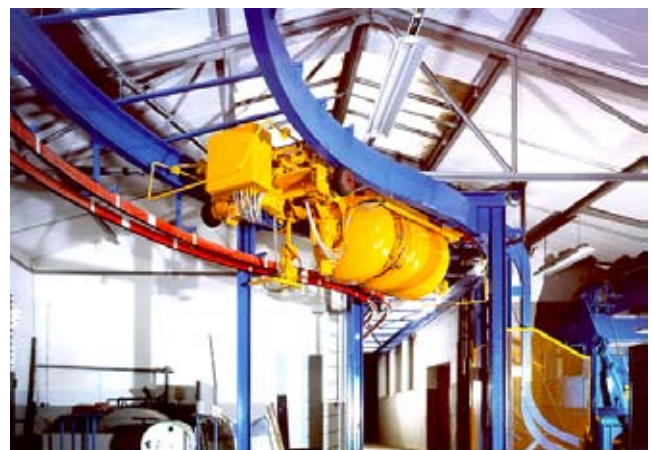
Feed and control of a concrete skipper
