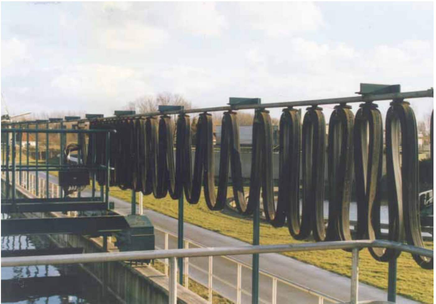
AKAPP Festoon installation with flat cables at a water purification plant
